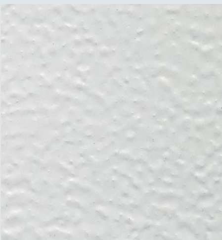
Stucco-textured surface finishes
